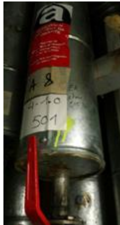
Joints mastic et calorifuges
