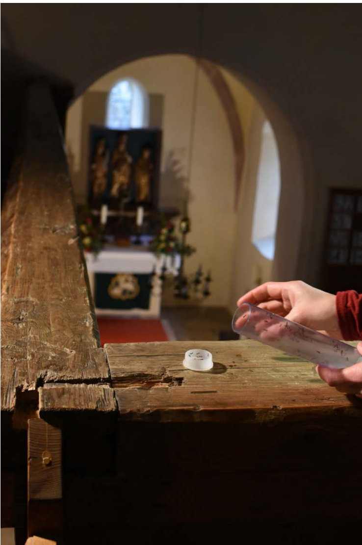
Figure 4: Release of Spathius exarator Depending on the infestation level, four to ten units, each containing about 100 wasps are released at infested objects within the treated buildings.
