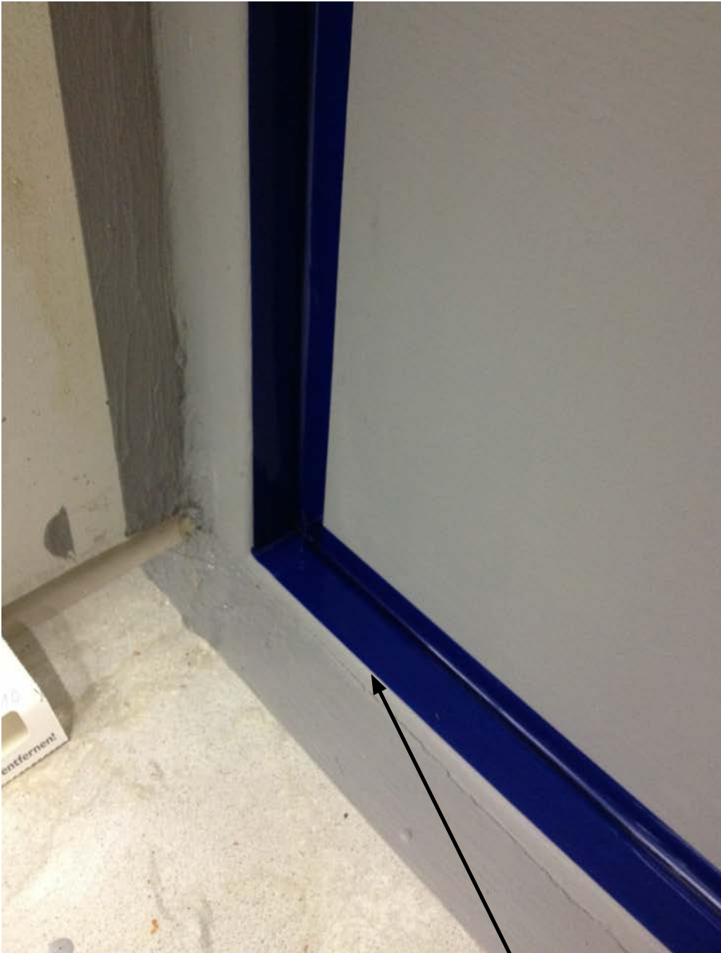
Fig. 7: Closed gaps between doors and doorframe with tape
